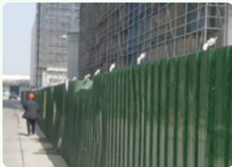
Spray dust removal facilities were added and bare soil was covered with dust screens at the construction site of Haiyang Polyamide
